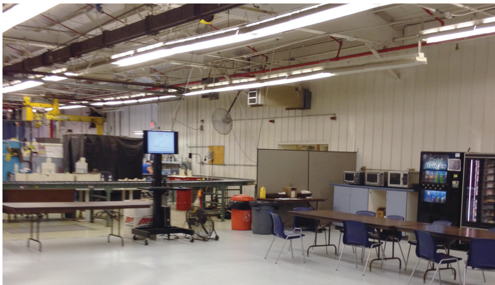
Many energy efficiency upgrades were made to the Triumph Thermal Systems facility in Tiffin
