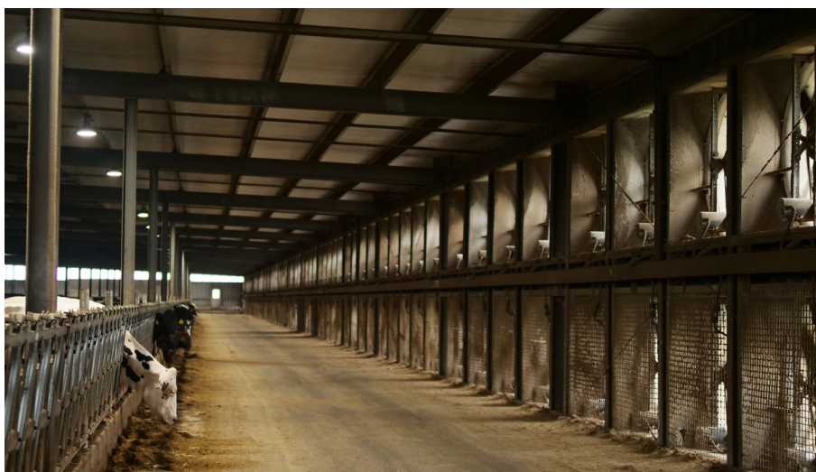
South Fork Dairy's high-efficiency exhaust fans help keep the cows more comfortable
