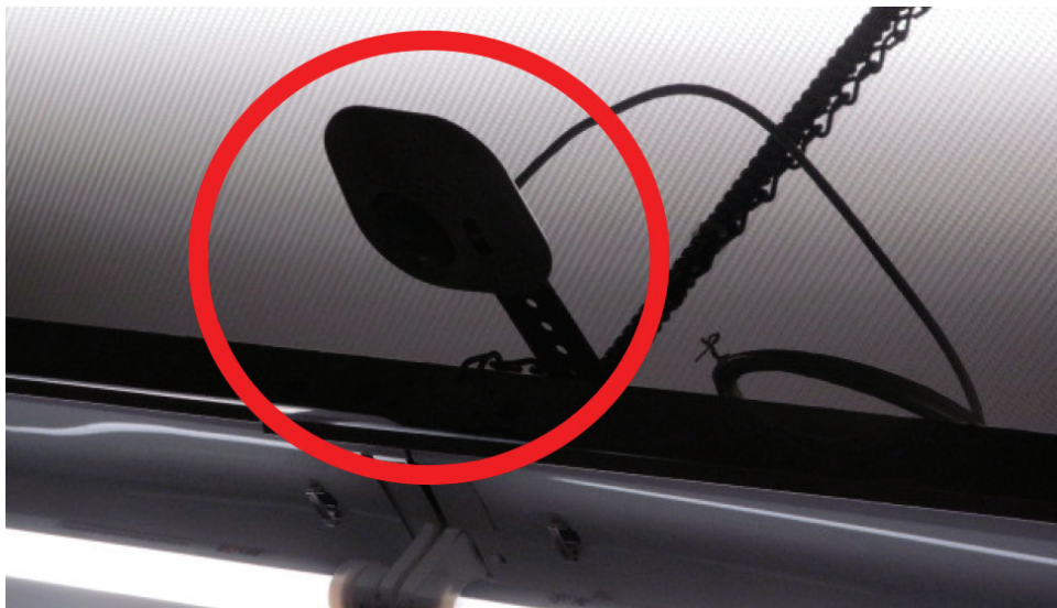
AT&T's lighting upgrade included installation of lighting sensors throughout the three facilities
